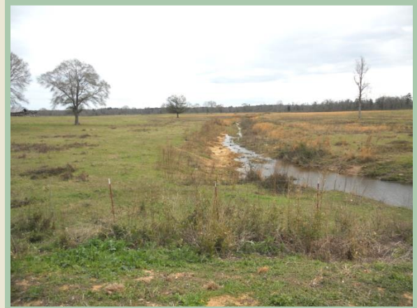
Figure 21: Stream Crossing for Cows without Fencing or BMPs
