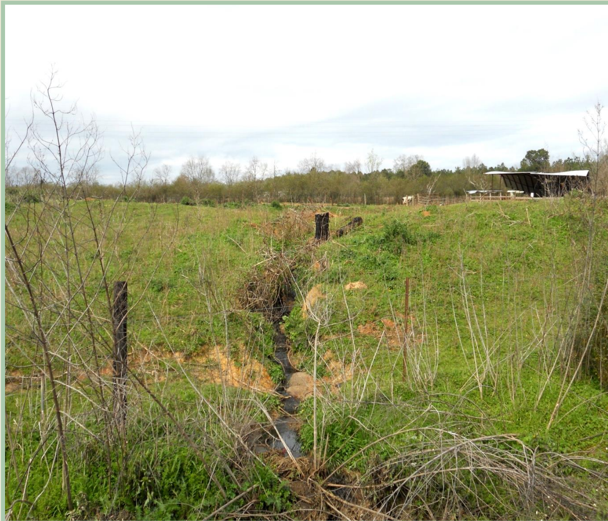
Figure 19: Waste Waters flowing from the Lagoon's Spillway
