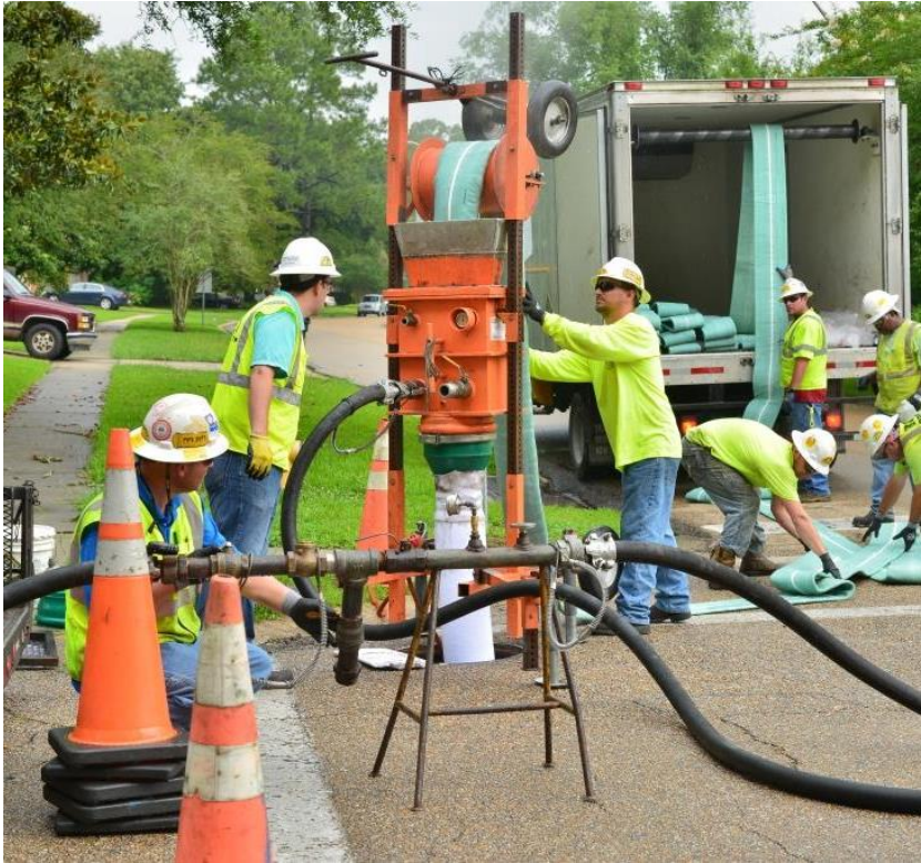
Connection to Sewerage: Regionalization
