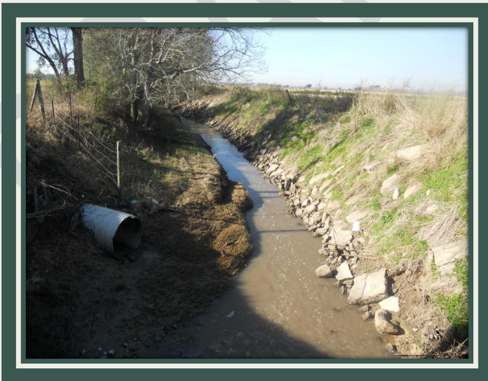
Site 5: Hoffpauir at Unnamed Indian Bayou Tributary Downstream
