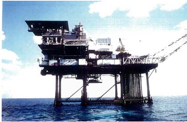
PHOTOGRAPH 4 – Lower Right Eugene Island 361A reference platform.
