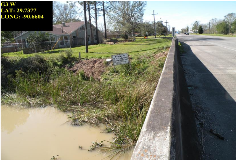
G3 Bridge at Hwy 1 over Theriot Canal
