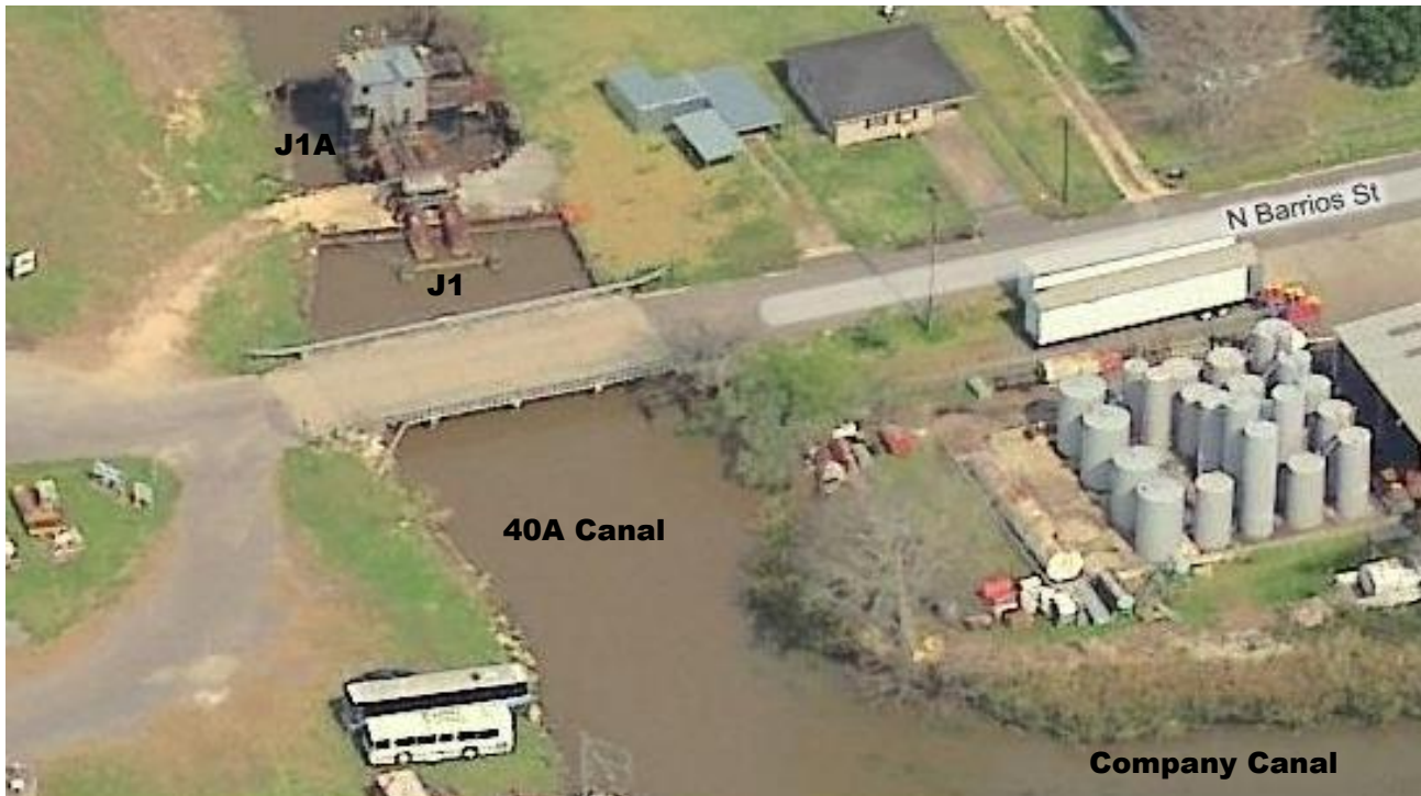
J1 & J1A - Virtual Earth Image of pump station at the 40 A Canal to the Company Canal, Lockport
