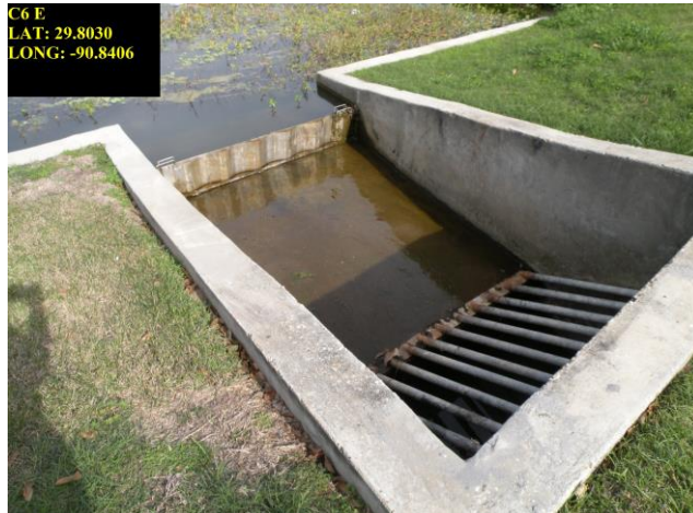
C6 The Lake drainage canal at control
