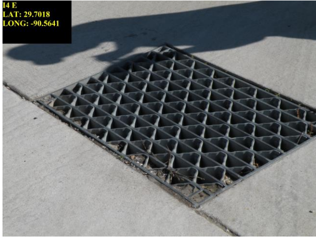
14 Culvert on Acadia Drive in Raceland
