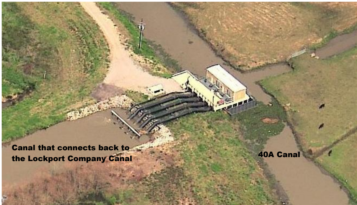
This very large forced drainage pump in the 40 Arpent Canal drains all of the pasture land adjacent to the Mar – Romy subdivision south of Lockport, and any drainage from the subdivision also. This pump drains this entire area into a canal that connects back to the Lockport Company Canal, which can directly impact Bayou Lafourche.
