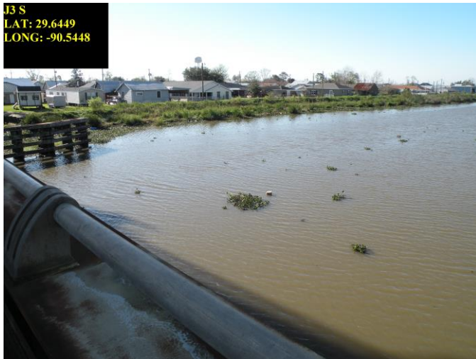
J3 -Bridge over Company Canal, Lockport
