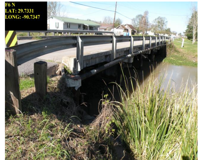
F6 Bridge 40 A on St. Charles Bypass Rd.
