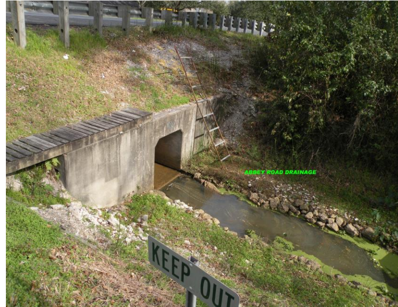
Abby Canal on Hwy 308 to B. Lafourche at LA 1385 bridge
