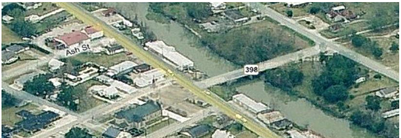
Virtual Earth Image of Site A1 bridge
