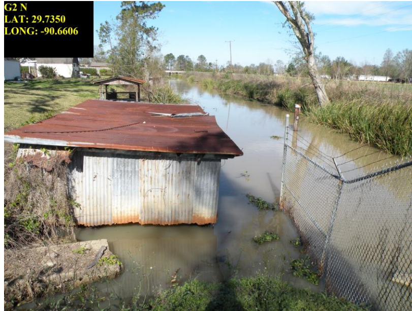
G2 Theriot Canal gate on B. Lafourche side
