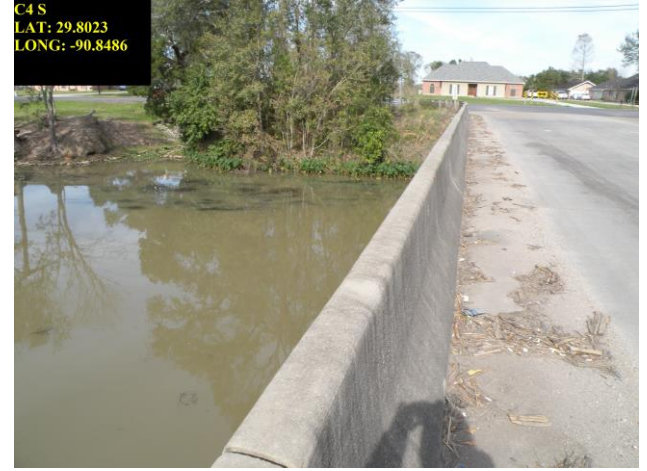
C4 Hwy 3185 bridge downstream
