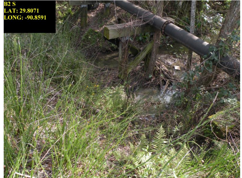
*B2 Degravel Canal at Hwy 1 ("Hot Spot")
