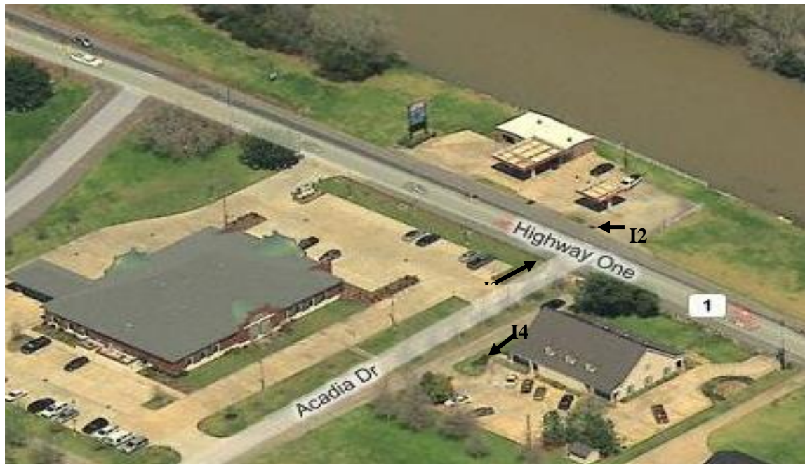
Virtual Earth Image of I2, I3, and I4 at Hwy 1 and Acadia Road
