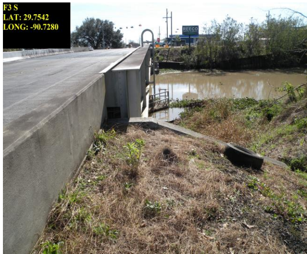
F3 B. Lafourche Bridge at St. Charles
