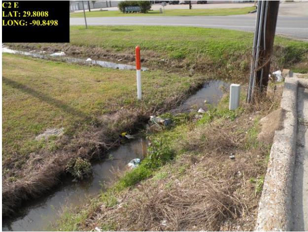
C2 Hwy 3185 apartments behind Rouse's shopping center
