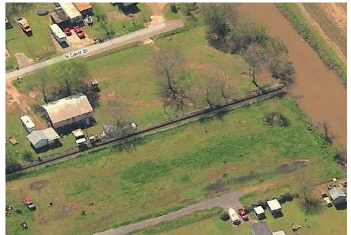
J2- Virtual Earth Image of Lockport Heights drainage ditch into the 40 Arpent Canal
