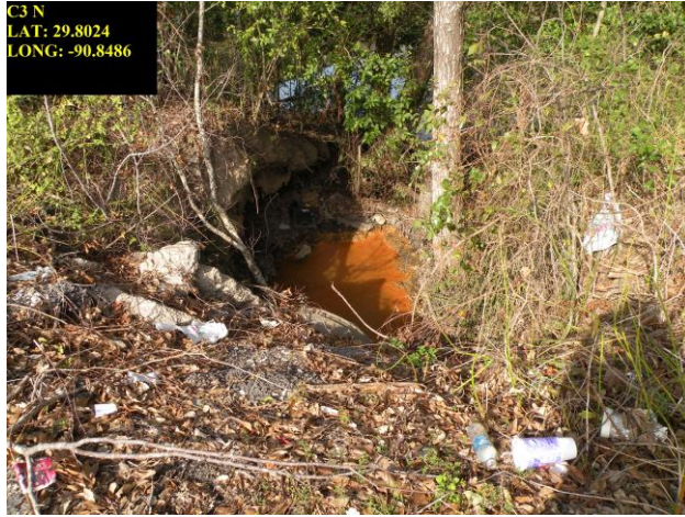
C3 Hwy 3185 culvert at B. Lafourche 3185 bridge
