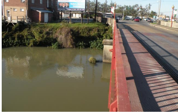
D3 B. Lafourche Bridge at Hwy 20
