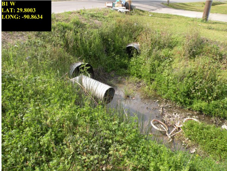
B1 Degravel Canal at Parish Road
