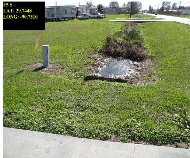
F5 321 St Charles Bypass (F4 for ditch near Hwy 1 not located)
