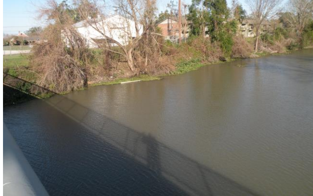
D6 B. Lafourche Pedestrian Bridge
