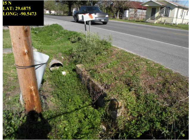
15 Culvert at 4926 LA Hwy 1, Mathews
