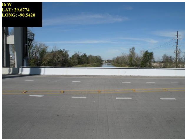
16 Bridge at Hwy 654 to Gheens (in Mathews)
