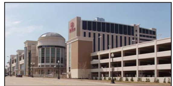
The completed Shreveport Convention Center.
