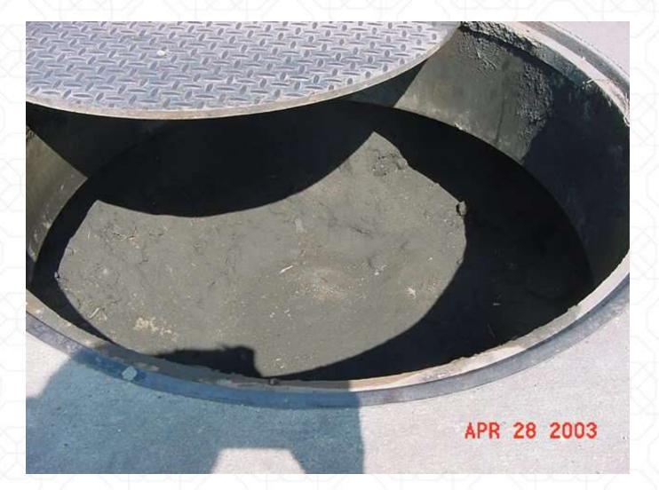
STP Sumps must have liquid tight sides and bottoms and be maintained free of storm water and debris
