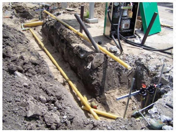
UDC Sumps required when installing new dispensers at existing facilities where new piping is added
