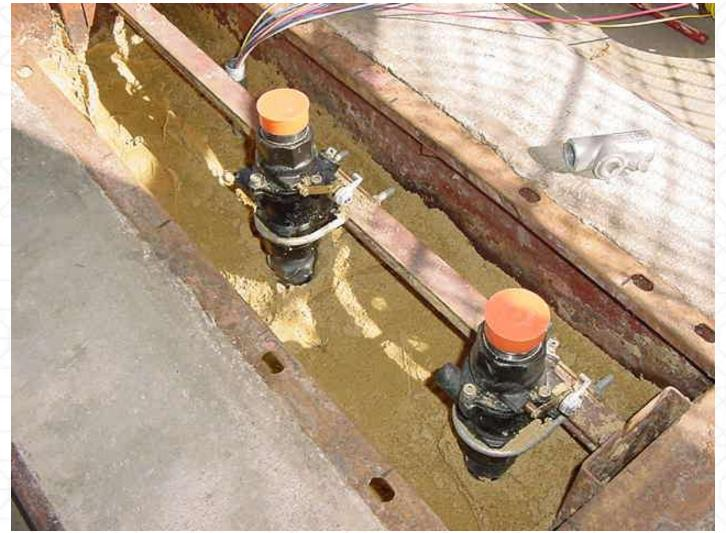
UDC Sumps not required when replacing dispenser only when nothing below the shear value is replaced
