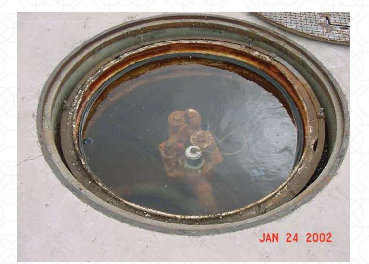
STP Sumps must have liquid tight sides and bottoms and be maintained free of storm water and debris
