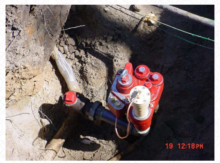
STP Sumps required when installing new STP (STP, housing and riser) at existing facilities where piping that connects STP to the existing piping is replaced
