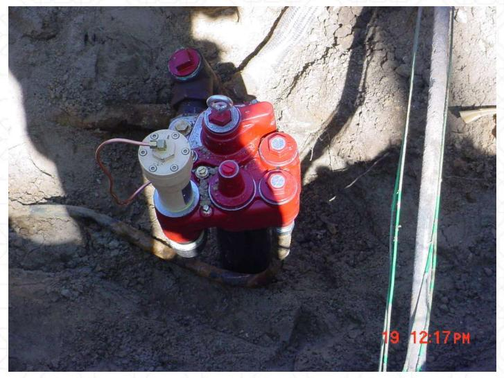
STP Sumps not required when installing new STP (STP, housing and riser) at existing facilities where no piping is replaced
