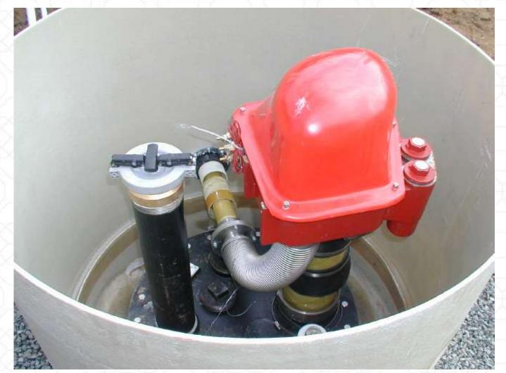
Installing built-in secondary containment (DW STP housing and DW flex connector) would not require a containment sump
