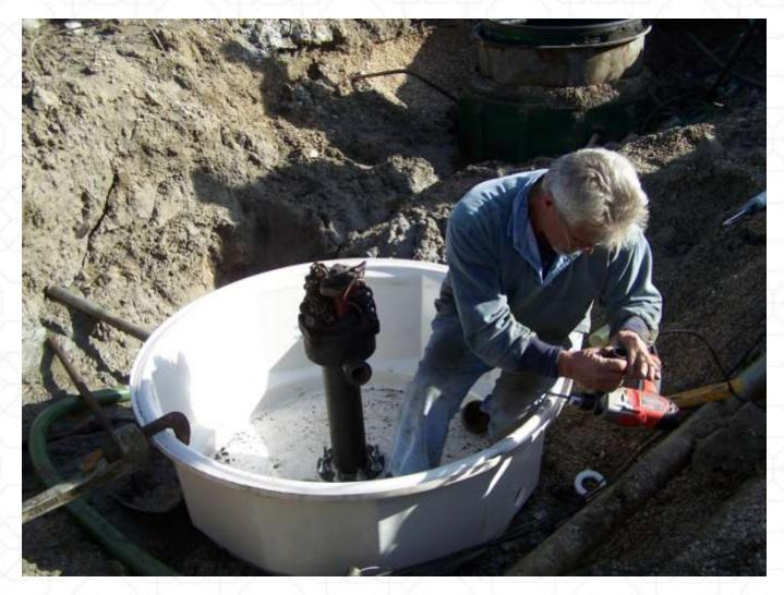
STP Sumps required when installing new STP (STP, housing and riser) at existing facilities where new piping is added
