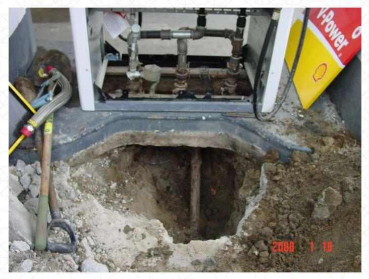
UDC Sumps required when replacing dispenser where new piping or components below the shear valve are replaced
