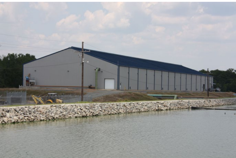
West Monroe Waste Treatment plant
