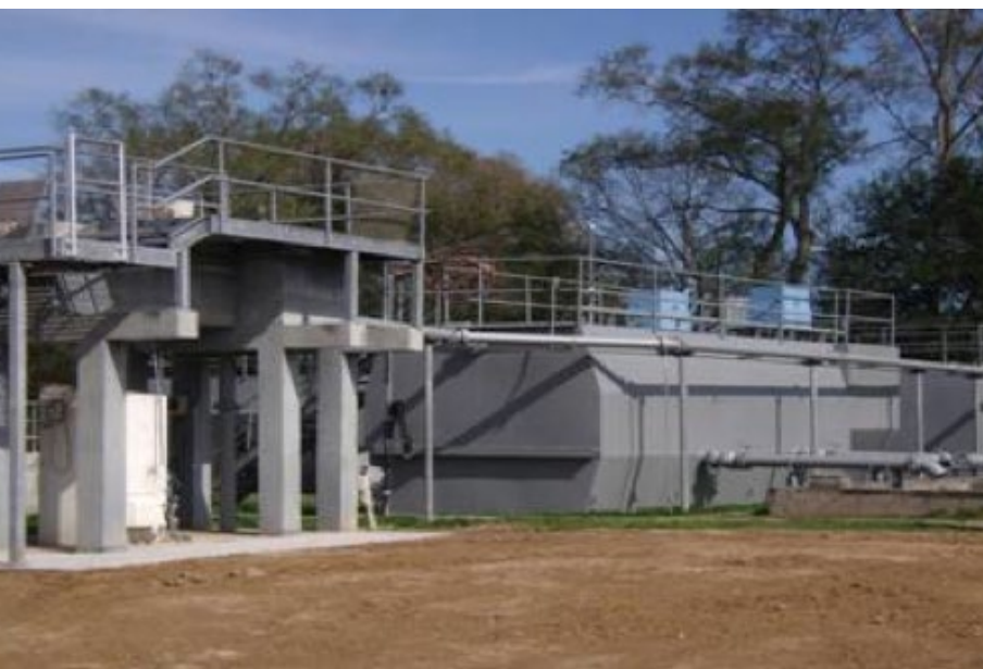
Maurice is using a Biolac System, which is an extended aeration process for waste treatment
