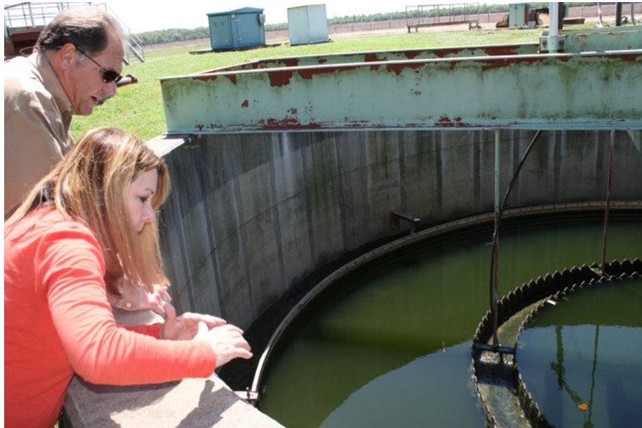
DEQ Environmental Scientists Wayne Slater (left) and Joette Kenaley inspect a water clarification unit at the wastewater treatment plant in Cheneyville
