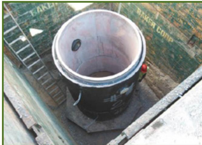
*A wet well under construction at the Mansura project.*
