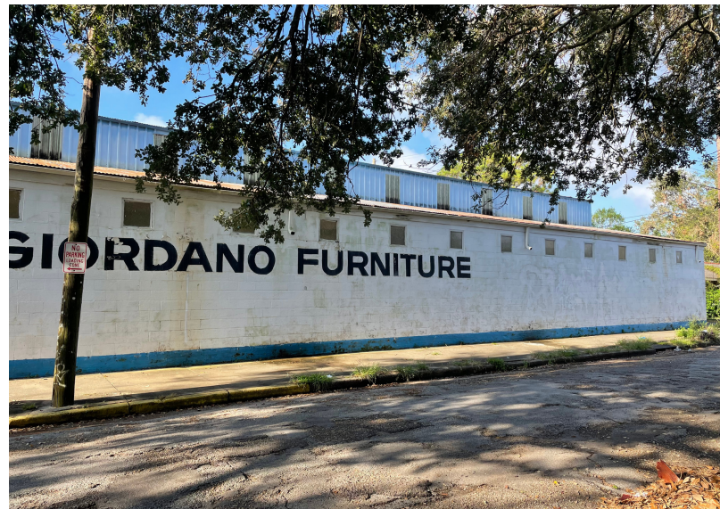
The former Giordano Furniture Warehouse is the future home of Beanlandia. Redevelopment activities are being conducted in conjunction with environmental assessment activities.
