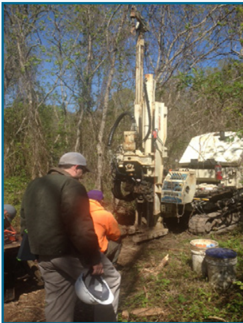
Destin Hooks and remediation contractors stand near a boring machine that is being readied for startup. The machine is used to extract soil samples in four-foot increments. With the boring completed, screen and tubing can be inserted to depth and groundwater sampled.
