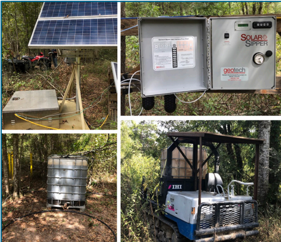
As solar panels power the sipping unit, the product is extracted from the well (indicated by the yellow pipes in the background) and sent via a tube into a holding tank (foreground) at the site. A regulator on the tank triggers when it's full. Once full, the product in the tank is emptied into a mobile container unit affixed to a Marooka IC30 tracked vehicle (right), which transports the product offsite to a staging point where it's shipped to Texas for proper disposal. The process repeats and will continue until sampling results indicate compliance with health and environmental standards.
