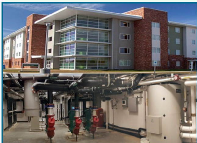
2019 Award Recipient - Southeastern Louisiana University's newest residence halls, Ascension Hall and Twelve Oaks Hall, draw from 220 geothermal wells situated 300 feet underground to heat and cool 556 rooms.
