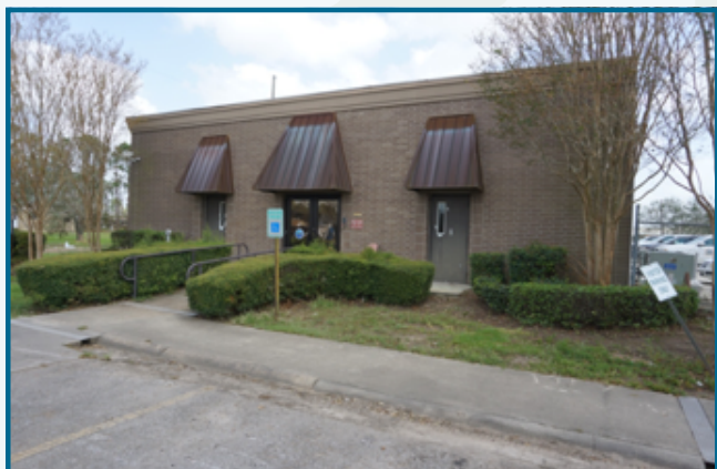
SWRO offices suffered little damage from Hurricane Laura.
