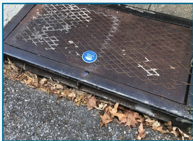
A storm drain marker serves as a reminder to keep this drain debris-free, but it's up to everyone to check and clear their local drain to prevent flooding.
