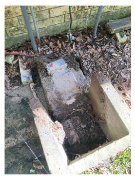
Figure 2 - Aerator covered in ants and not working
