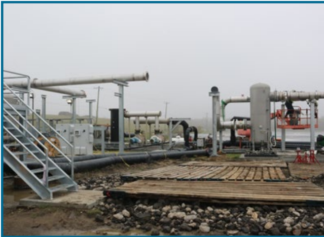
The gas processing plant at River Birch
