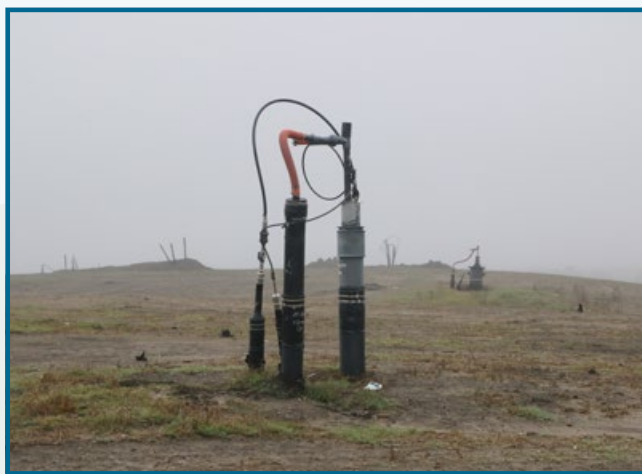
Gas collection points at River Birch landfill
