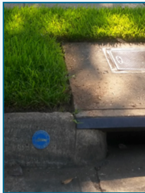
Blue discs are attached next to storm drains to inform the public that illegal dumping can have a direct effect on the waterway.
