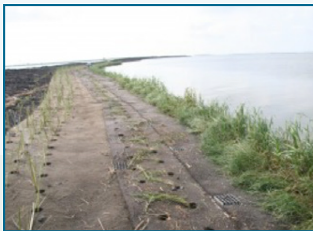
Photo by Martin Ecosystems Vegetated EcoShield™ is infused with native plant species and placed along shorelines to support and strengthen the existing ecosystem.
