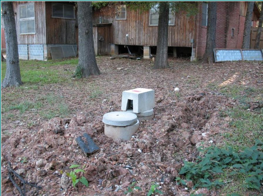
Upgraded system to a mechanical plant and removed direct discharge line to Cross Lake.
