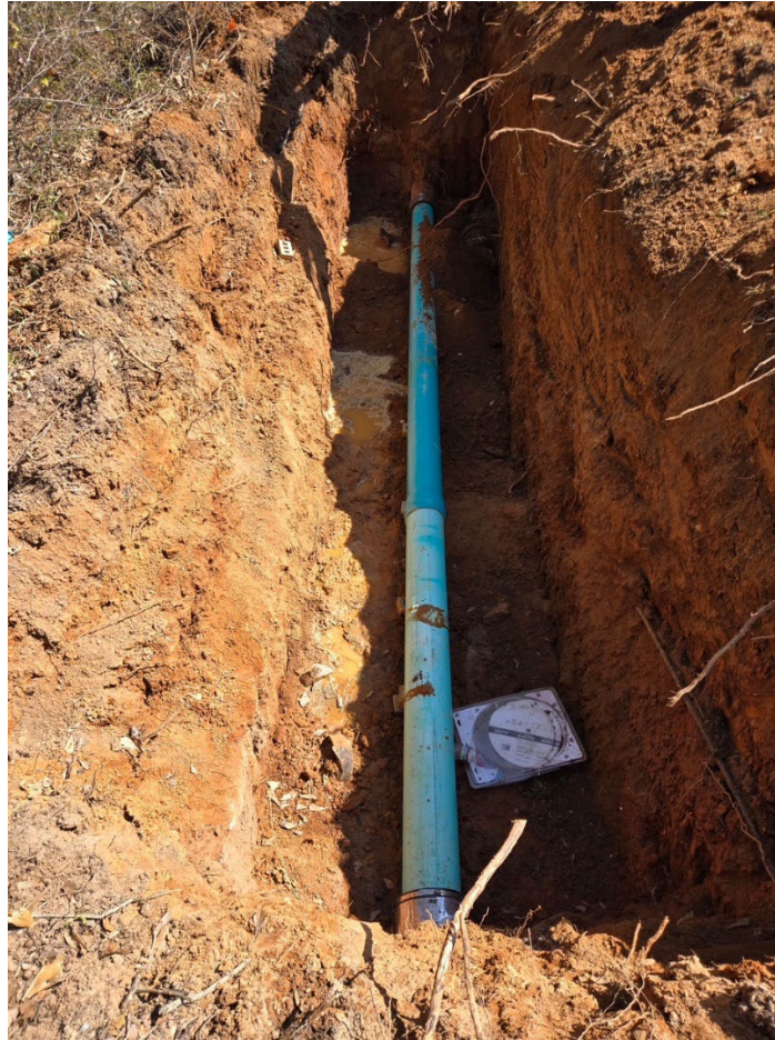
Picture 5: Typical Gravity Sewer Point Repair Project
