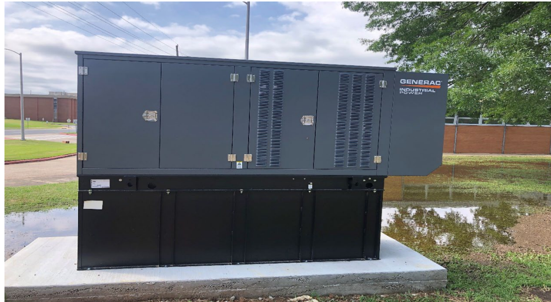
Picture 1 – City of Grambling new generator installation
