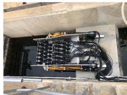
Picture 3: City of Shreveport UV Disinfection Bank
