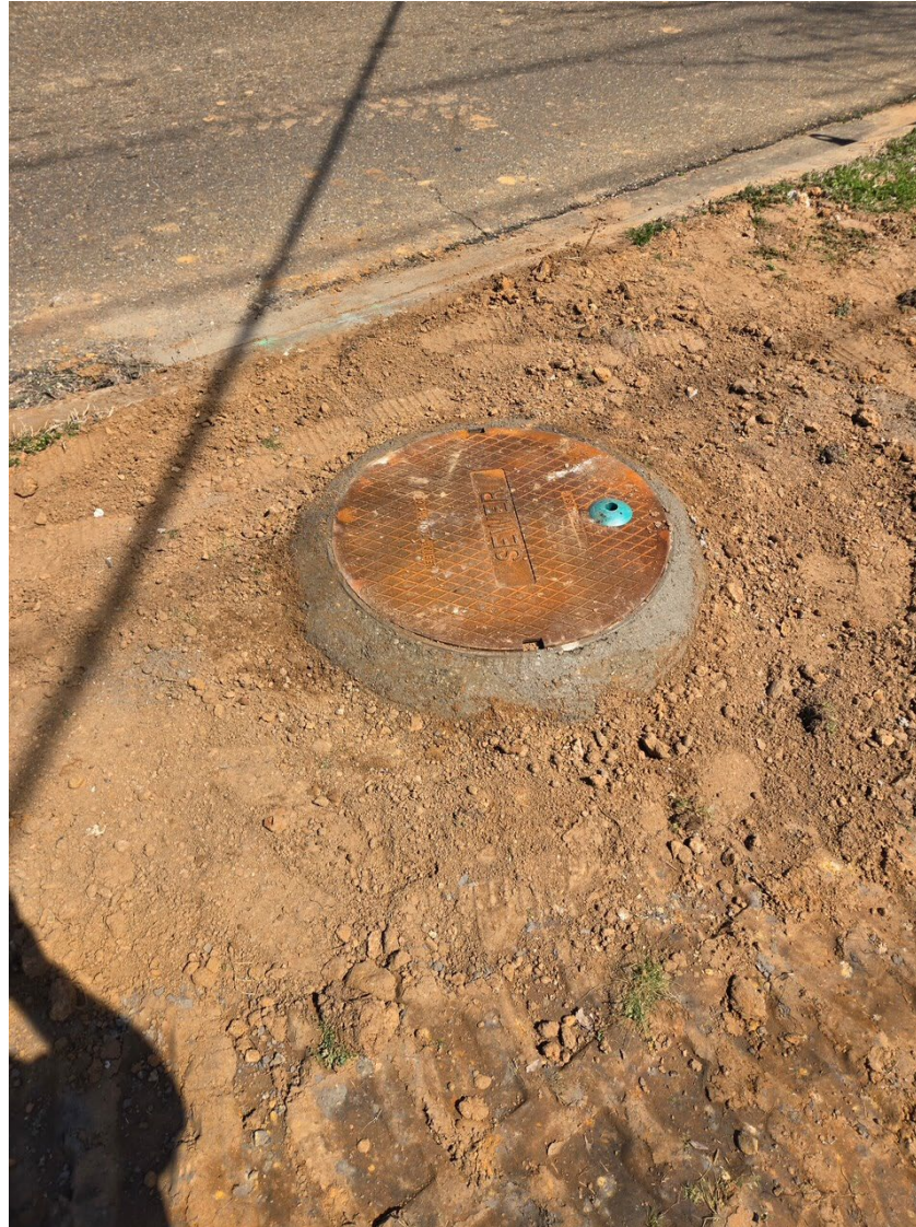
Picture 5 – Typical Manhole Rehabilitation Project
