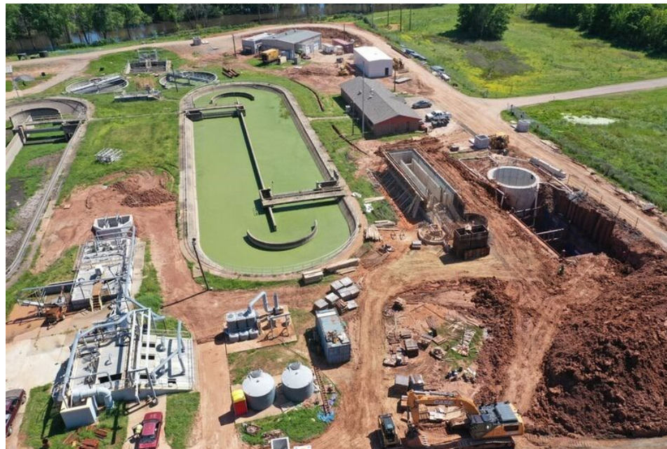
Picture 1 – WWTP Rehabilitation, Bossier City, LA
