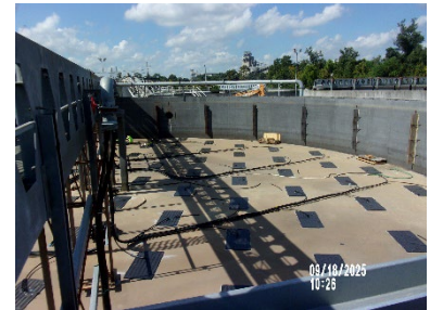
Picture 3 – Aeration Basin Rehabilitation, Destrehan, LA
