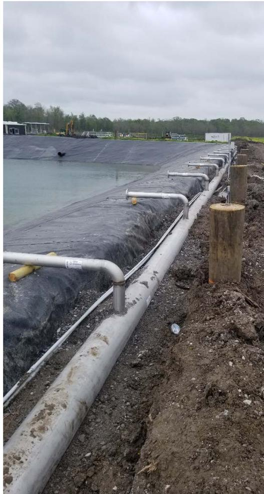
Picture 1: WWTP earthen aeration basin with liner and aeration piping
