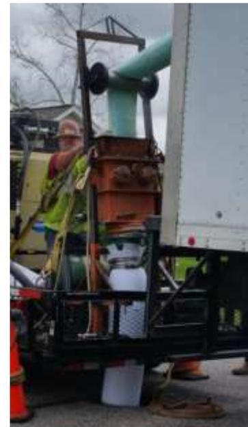
Picture 3: Contractor performing CIPP lining of sewer gravity main
