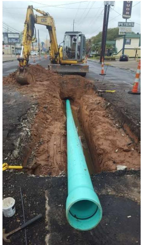
Picture 2: Collection system Rehabilitation – Pipe Removal and Replacement
