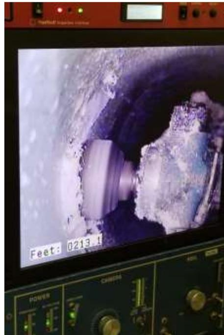
Picture 1: Contractor cutting out sewer gravity main CIPP lining to reconnect gravity service line.
